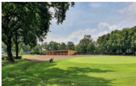
Neubau Driving Range.
